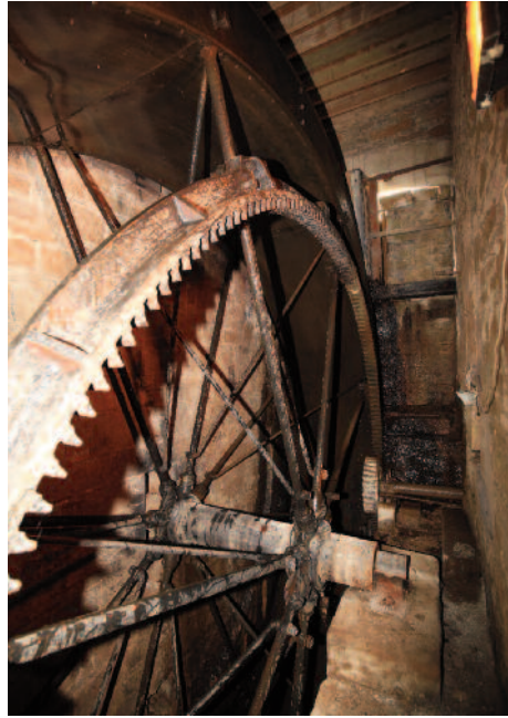
Fig. 1. All-iron suspension waterwheel at Dyan Mills, Caledon, County Tyrone, Northern Ireland, c. 1829.
