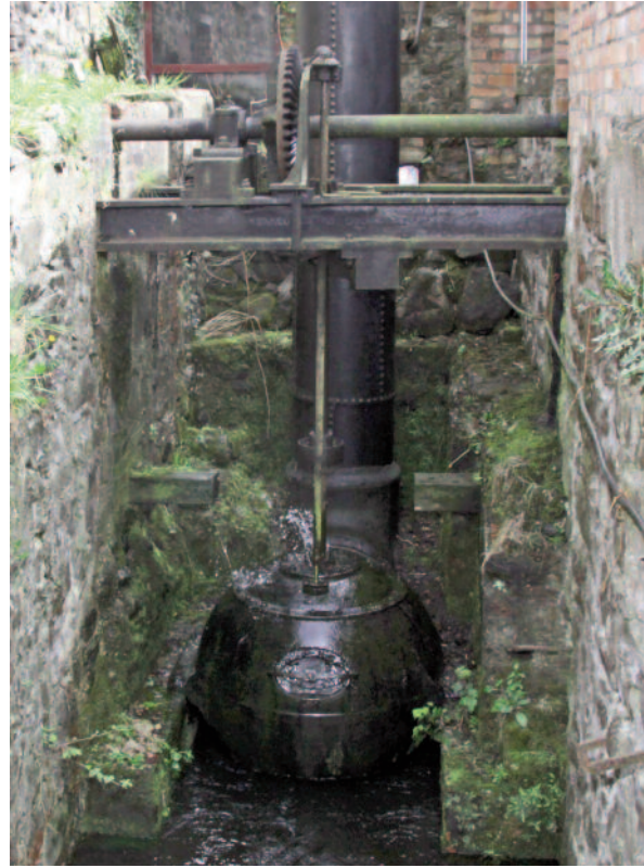
Fig. 5. 'Double' Leffel turbine, c. 1920, at Patterson's Spademills, Templepatrick, County Antrim.
