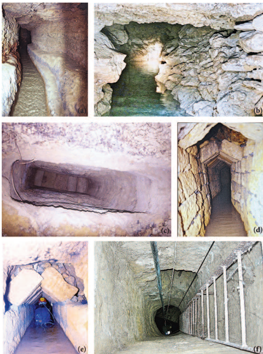
Fig. 8. Qanāts and wells in Palermo: a) Danisinni qanāt ; b) Scibene qanāt , with a dry-stone reinforcement wall; c) Senia well (Gesuitico basso senia at the Vignicella qanāt ); d) Corso Calatafimi basso qanāt . Roof covering and retaining wall in large calcarenite blocks; e) Maurigi qanāt , excavation in a trench covered with large clamped blocks of calcarenite with roof contrasting “buttonhole” shafts (“furnace mouth”); f) Well-shaft of the Cuba Soprana.
