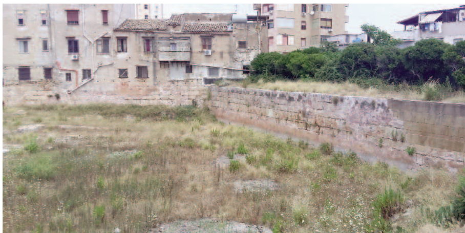
Fig. 14. Masonry dam of the Favara-Maredoce artificial lake.
