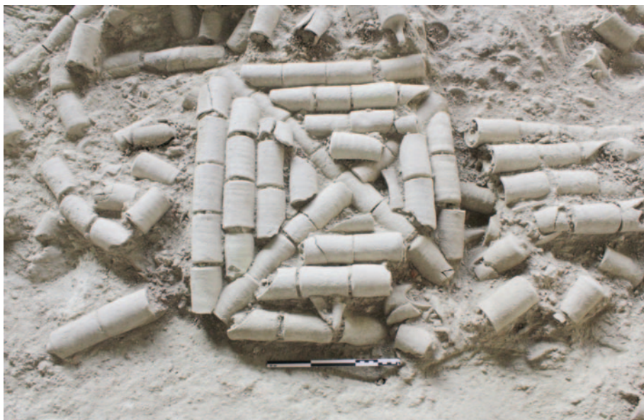
Fig. 7. Terracotta vaulting tubes keystone ( tubi fittili ).
