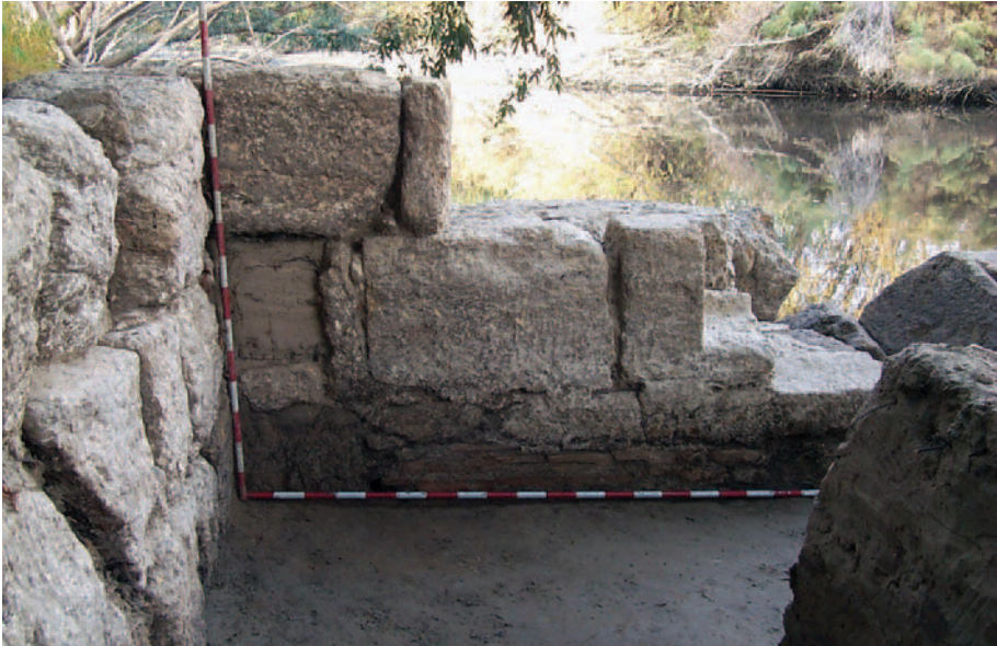
Fig. 12. La Palmosilla Baja . Building B. Detail of the construction techniques. Hole for a beam (left) and lintel of the entrance door (right) (S. García-Dils).
