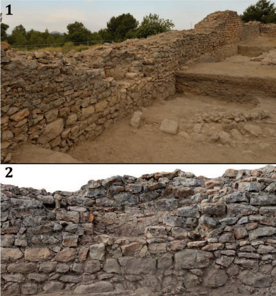
Fig. 7. Double staircase opened in the wall during the construction process. It is half-height, which requires a wooden ladder.
