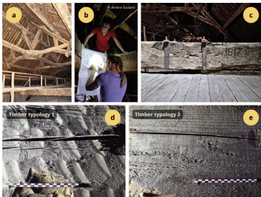
Fig. 9. The Cathedral of Montauban. (a) The roof structure; (b) sampling and recording trademarks; (c) evidence of restoration; (d) timber typology 1; (e) timber typology 2.
