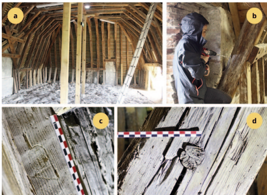
Fig. 6. The Episcopal Palace of Montauban. (a) The roof structure; (b) the sampling campaign; (c) trademarks on timber; (d) wooden peg with rope remnants.
